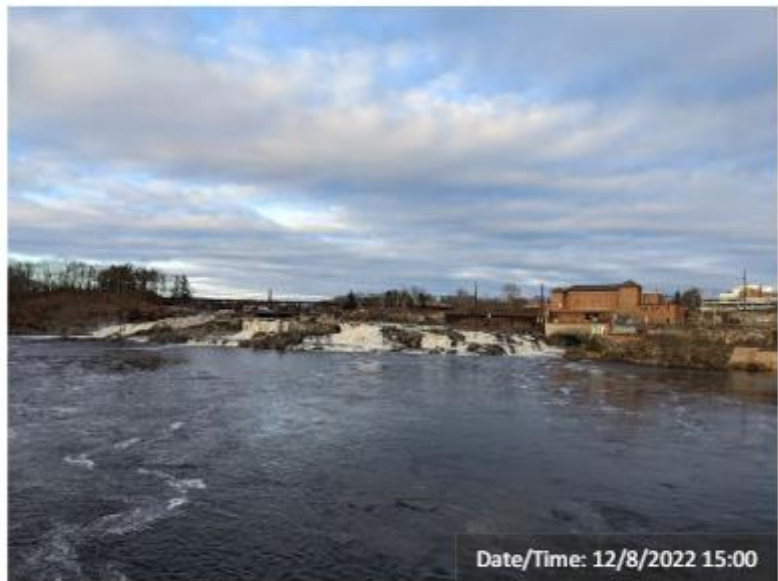
4,350 cfs spill, Dam 1 deflated, Headpond el. 168.29 ft
